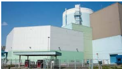
Nuclear Power Plant (NPP) Krško
