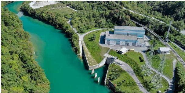
Hydro pump storage plant AVČE on the river SOČA
